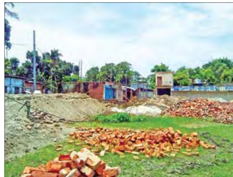
Bricks and sand kept ready for constructing buildings.
